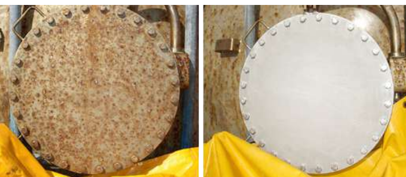
Before and after cleaning.
