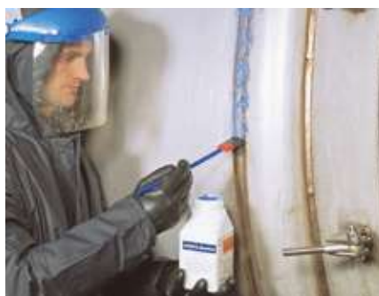
Photos showing the application of BlueOne™ Pickling Paste and the bright pickling result.
