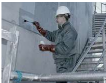
Photo: Site pickling with Gel 122, easy to apply thanks to its free flowing consistency
